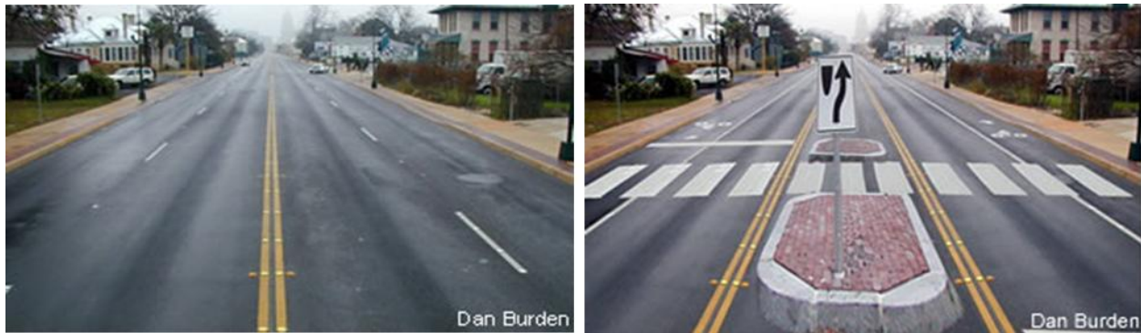
The classic road diet converts a four lane section to three lanes. In this scenario, the bike lane provides a buffer to pedestrians walking on the sidewalk adjacent to the curb.
